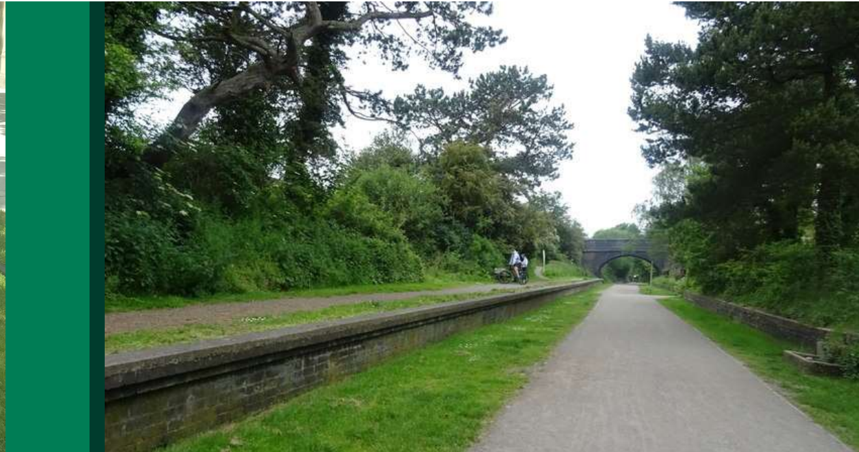
Segregated rural cycleway
