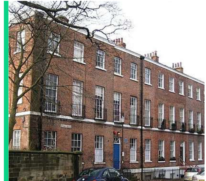
Brick Georgian facade
