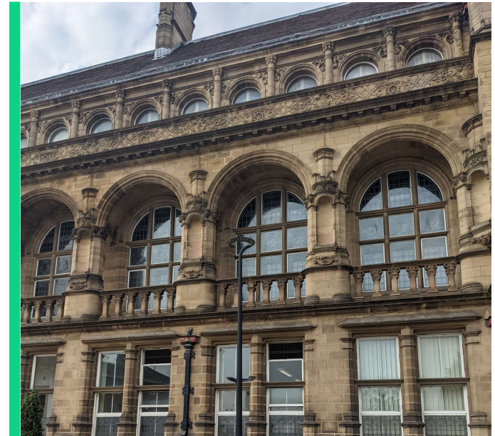
Civic architecture with intricate detail and texture
